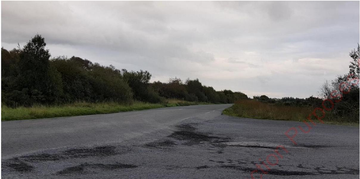
**Figure 12: Poor carriageway condition and loose debris at Site Access**
