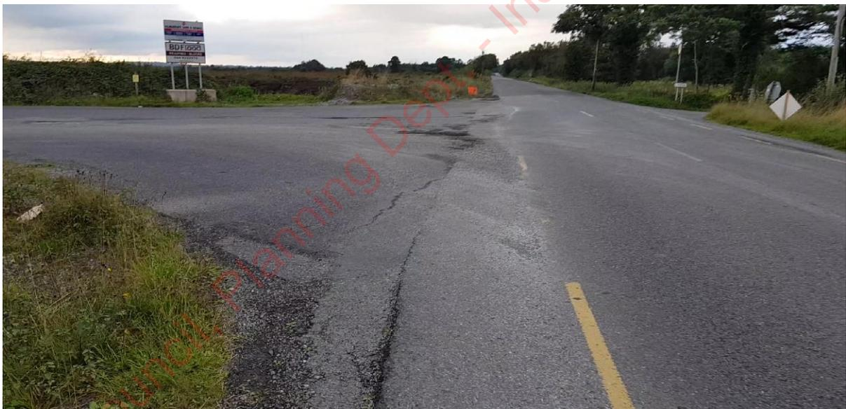
**Figure 11: Poor carriageway condition and loose debris at Site Access**
